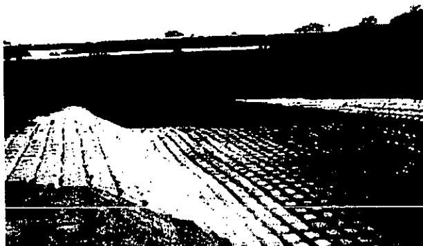
Figura 8.1.16 Tapete de concreto flexible.
